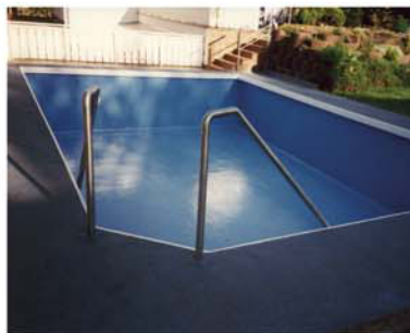
Schwimmbecken Swimming pools
