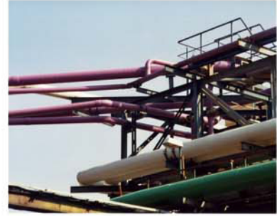
Rohrbrücke Pipeline bridge
